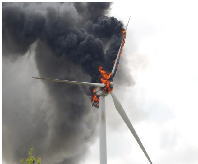
Figure 2 – Windpark Groß Eilstorf wind turbine fire [8]
